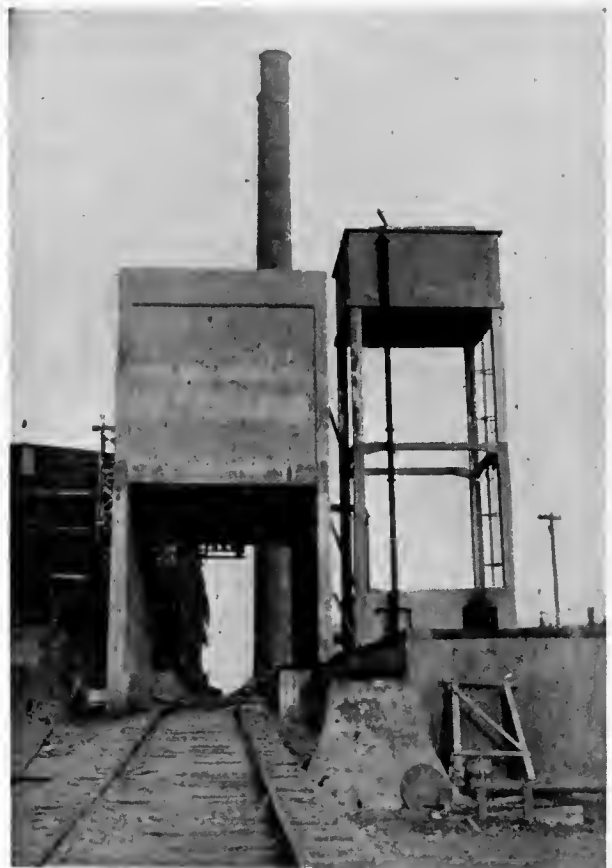
COKE QUENCHING PLANT
